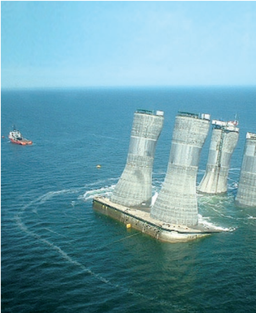
Photo: Aker Solutions marine operations
